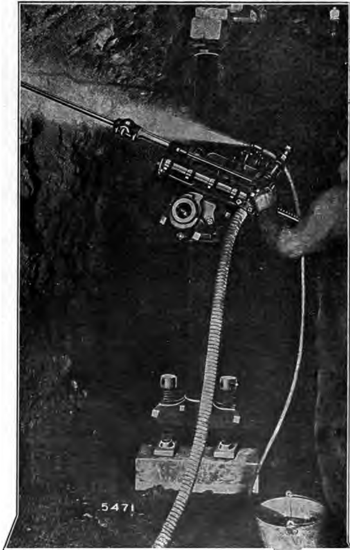
Fig. 34. Butterfly Drill with Water Spray.
